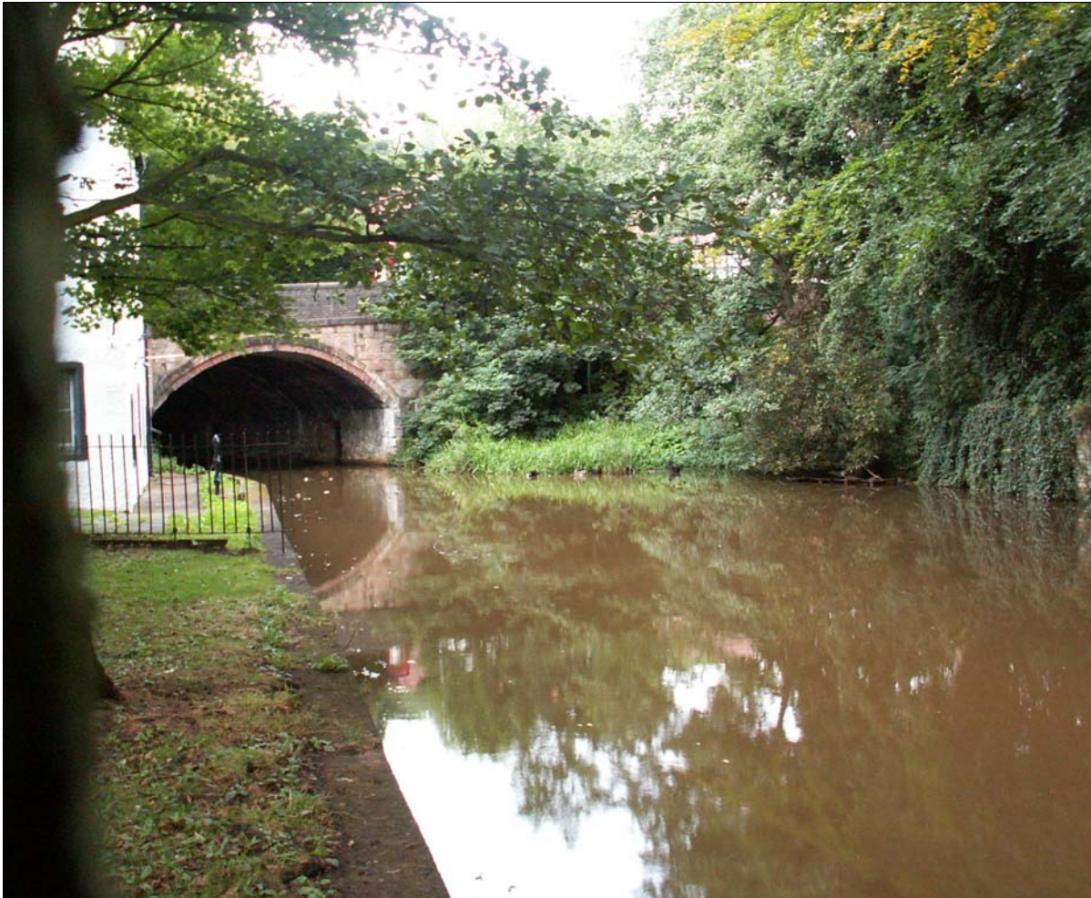
Above: Worsley Canal Basin (ref WB3).
